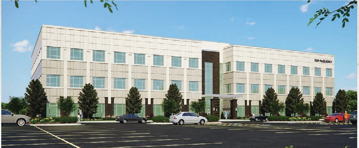
RSM McGladrey, a leading national CPA firm with offices throughout Illinois, is the anchor tenant at One Bell Valley Commons.
