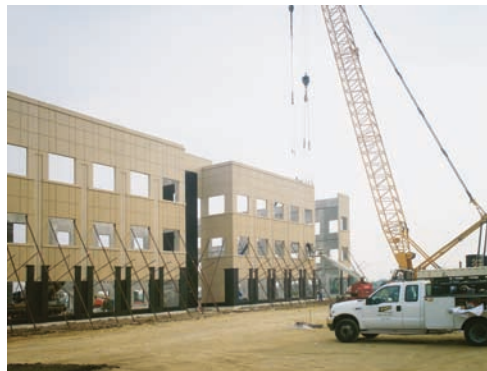
With the help of a 280-ton crane, the erection crew had the precast giants standing in just eight days!
